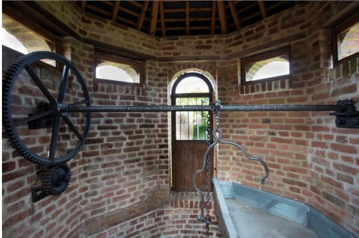
View of the inside and the mechanism's gear, pulley, bucket handle and reservoir © Département de la Seine-Maritime
