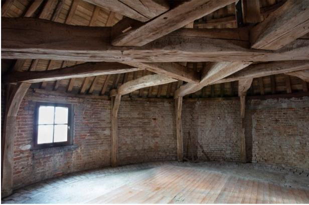
The roof structure is laid directly on the walls © Département de la Seine-Maritime
